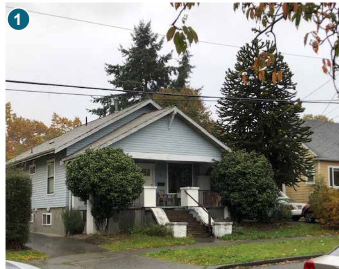
1 older homes near site, typical of area
