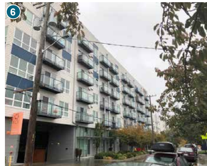
6 Koi - NW 54th Facade 6-story mixed-use residential
