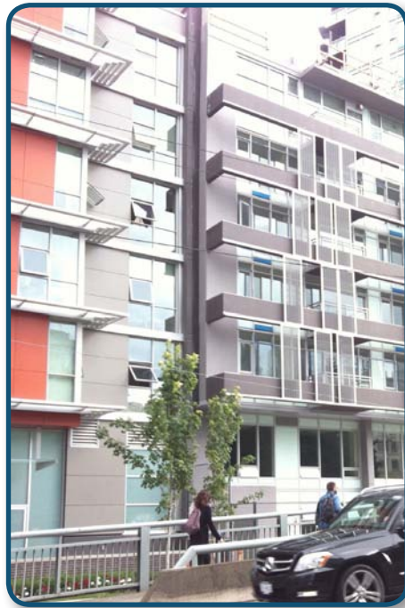
shading devices provide light control and variable pattern; variation of solid/ colored elements with lighter translucent ones creates a dynamic facade
