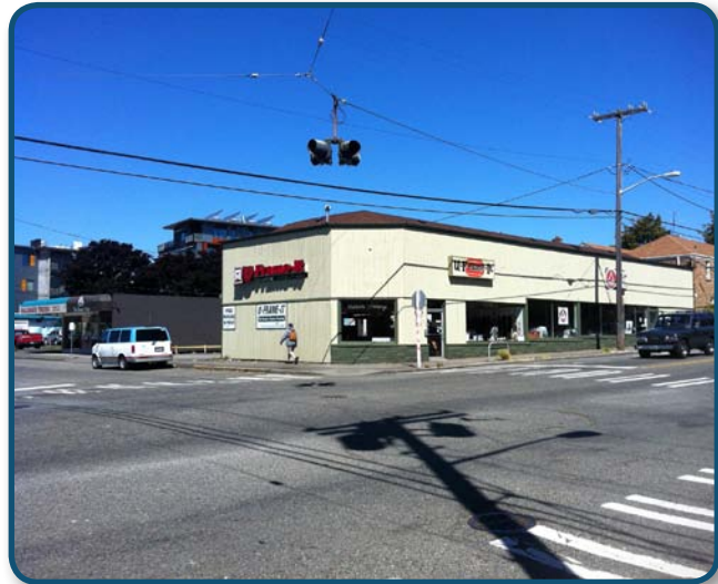
SE corner view
