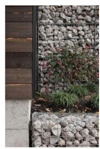
Integration of Gabion walls, concrete, cedar siding
