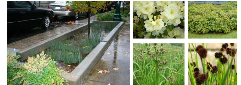
Bioretention planter with hard edge
