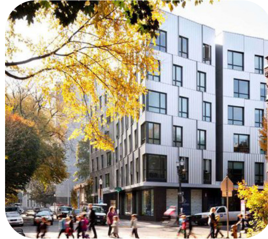
Architectural statement at the corner
