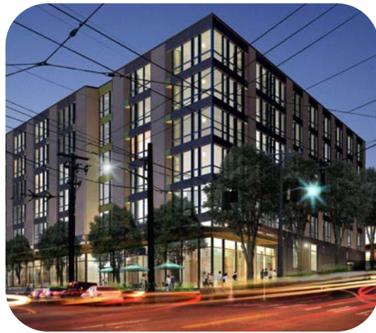
Commercial base with glazing
